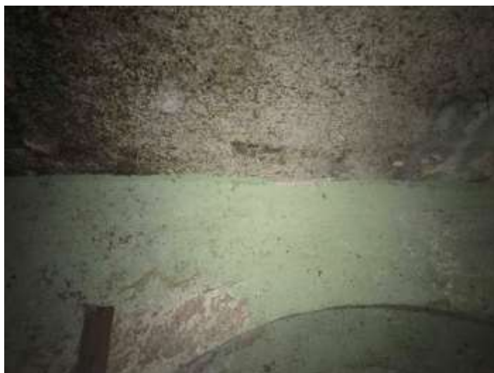
Slika 17: Strop in zidovi (Detmar, 7. 2. 2020)
